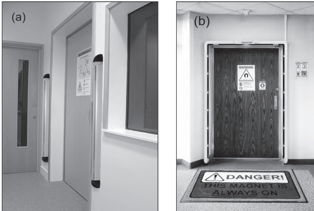
Figure 6. Examples of entryway or portal-type ferromagnetic detection systems. (a) Photograph courtesy of Metrasens, Ltd. (b) Photograph courtesy of Kopp Development, Inc.
