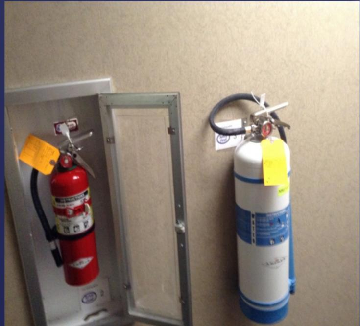
Both of these fire extinguishers were installed in the MR control room (Zone 3) of a MRI suite, one is **MR Conditional**, the other is **MR Unsafe**. This represents a potential MR safety risk!
